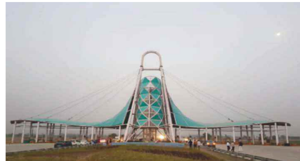
▶ DELHI EASTERN PERIPHERAL TOLL PLAZA
